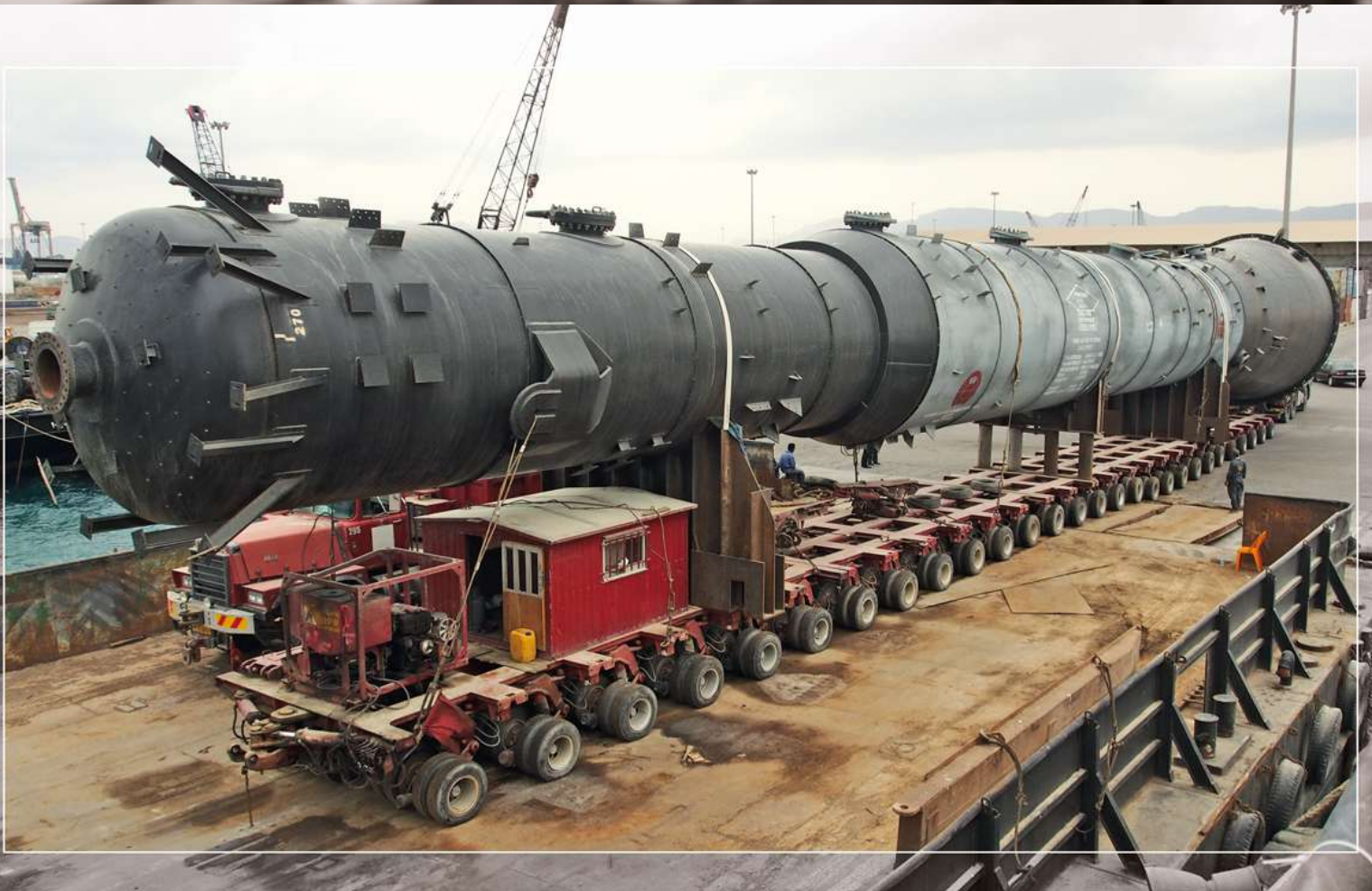
Design, Manufacturing and Installation of Refinery Towers
